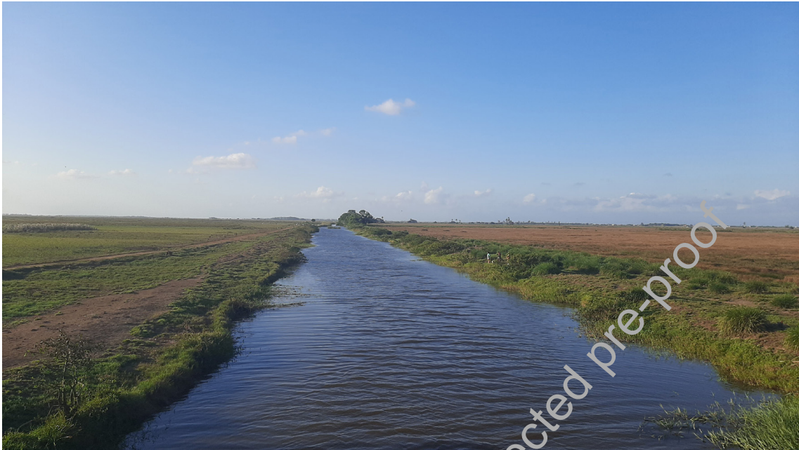
FIGURE 6. Drainage channel, downstream view near Suruaca Lagoon, accessed via ES-010, municipality of Linhares (Photo by Marcelo Parente Henriques, 2025).
