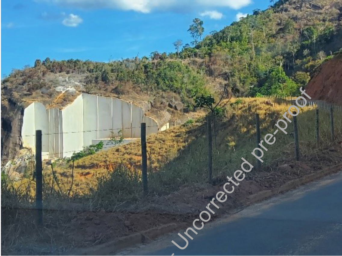
FIGURE 20. Extraction of dimension stone blocks in the western region of the municipality of Linhares.
